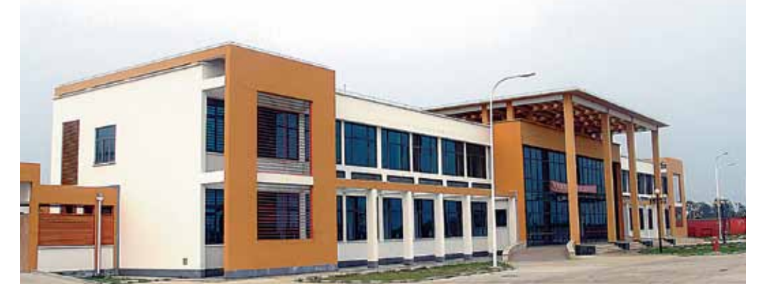
OYO hospital built by Beijing Uni-Construction Group.
